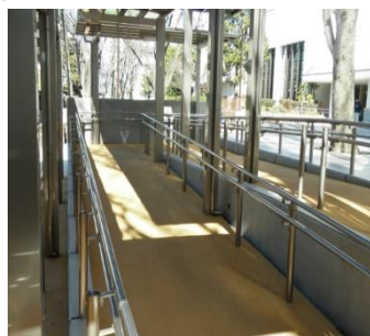
<Facility entrance renovated to install a slope>[2]
