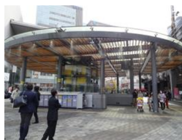
<Creation of cool areas>[2] Dry mist cooling system and heat ray reflection film
