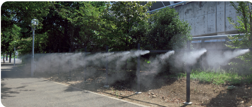
Dry mist cooling system at Tokyo Stadium
