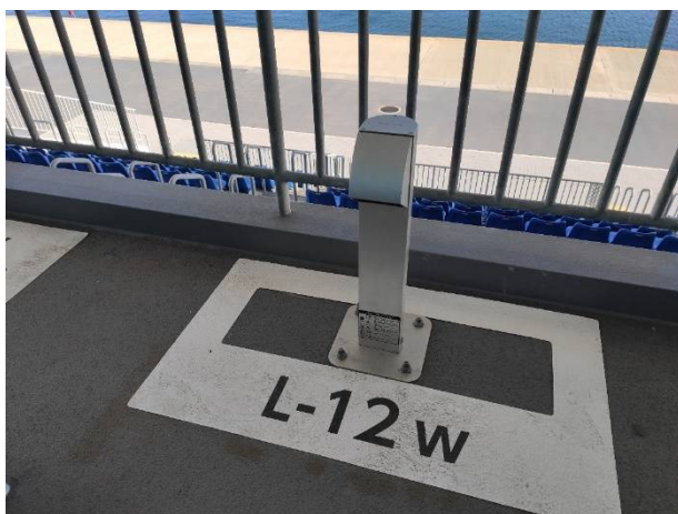
<Electric outlet for wheelchair battery charging>
