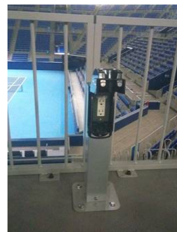
<Electric outlet for wheelchair battery charging>
