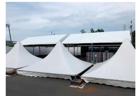
Measures to prevent temporary construction from becoming flying debris
