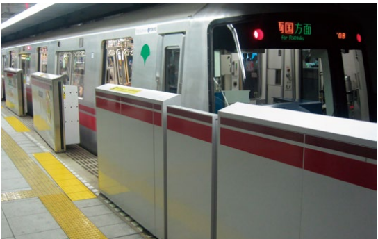
Installation of platform doors
