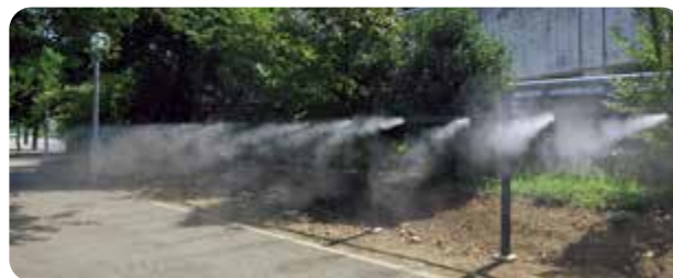
Dry mist cooling system at Tokyo Stadium
