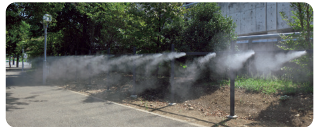
Dry mist cooling system at Tokyo Stadium
