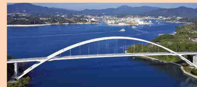
Kesenuma-Oshima Ohashi Bridge - Opened
