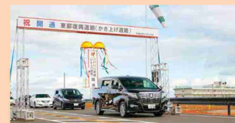
Eastern Reconstruction Road - Opened
