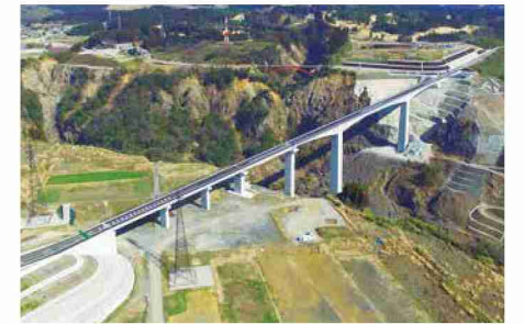
Shin Aso Ohashi Bridge (Opened March 2021)
